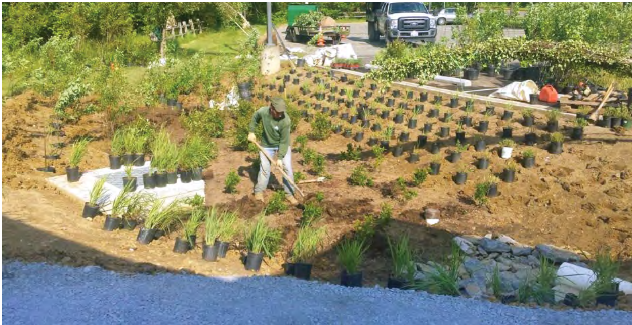
Figure 23: Stormwater infrastructure construction (Source: http://thecleanwaterpartnership.com )
